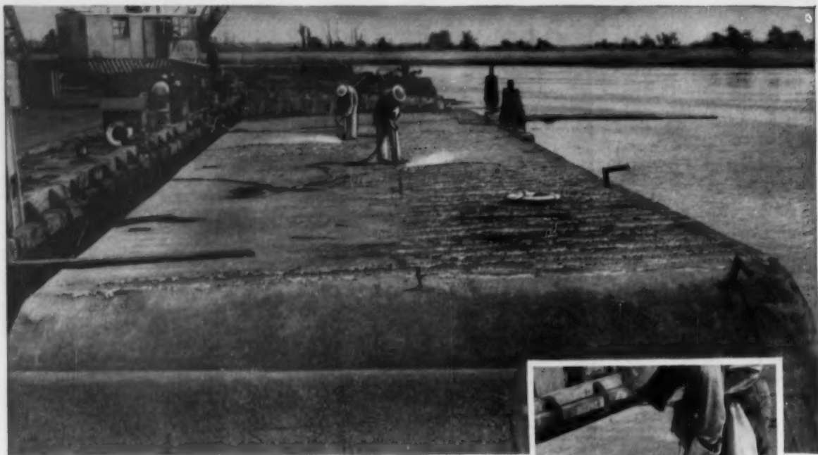
This C-51 deseaming blowpipe opens transverse plate welds in steel barge bottoms 7 times faster than the previously used process.
